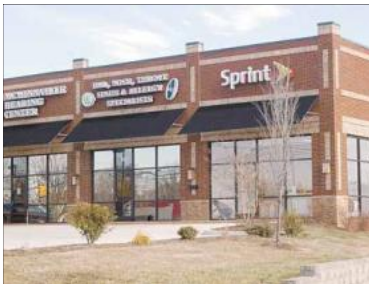
Renovation work is taking place inside the old Sprint store on Chancery Street near Rite Aid. Property owner Bobby Kirby says the building will be the site of a home health agency expected to open in March.
